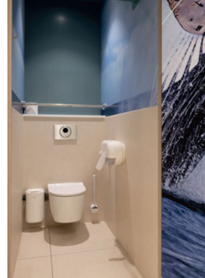
↑ Geberit ONE WC suite with TurboFlush and touchless automatic flush actuation means less cleaning work.
